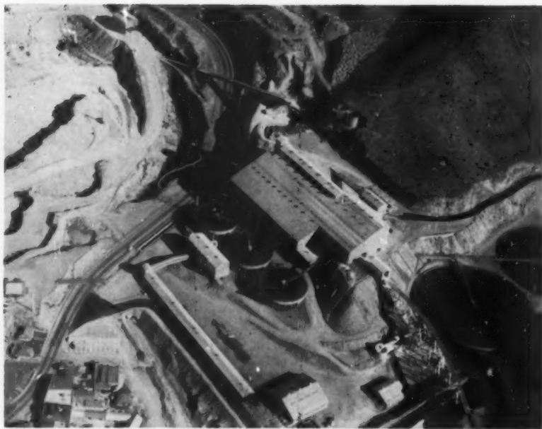
AERIAL VIEW of Lavender Pit mill shows pit and crusher (top left), and U. S. Route 80 winding under overhead belt conveyor going to the 12,000 ton per day concentrator.
